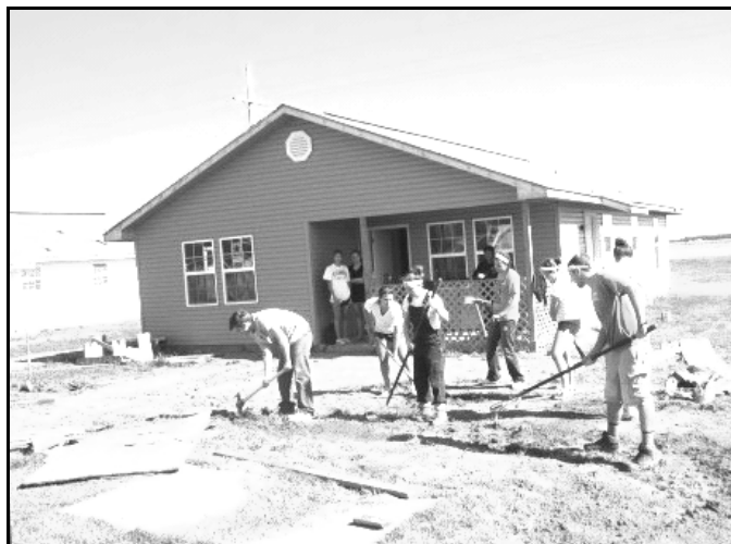
Villanova students hard at work outside Habitat House #37.
