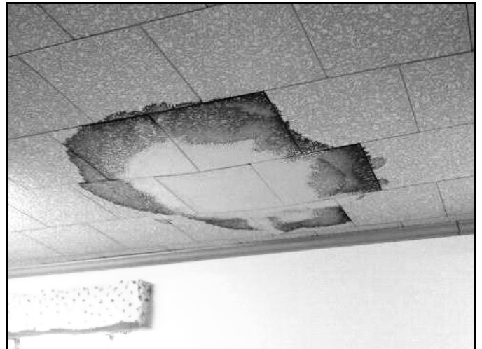
Leak in the office ceiling.
