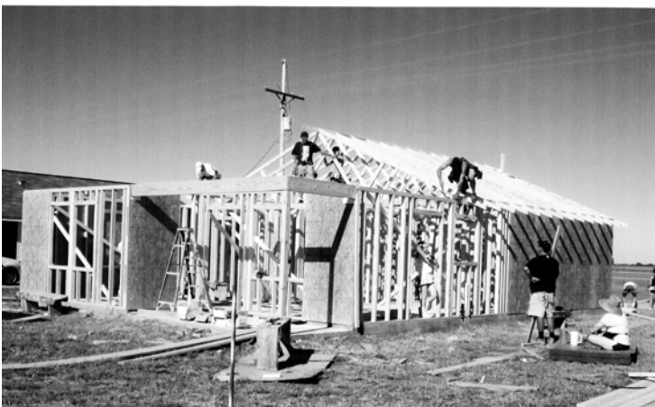
Another Habitat home under construction in Tutwiler.
