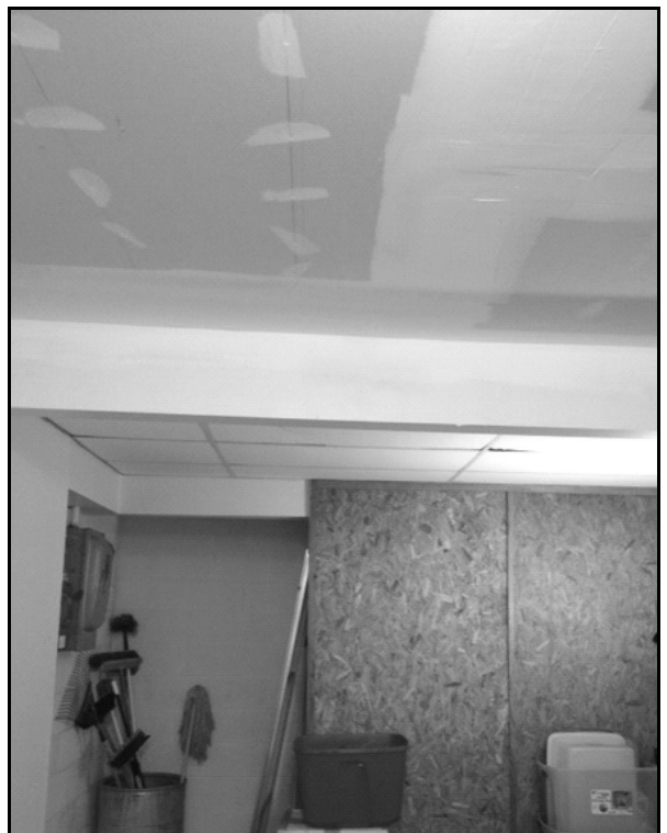
Ceiling repairs at the Bargain Barn made by the Sheil Center workers after-rain damage. (See 'Rain, rain...' page 2)
