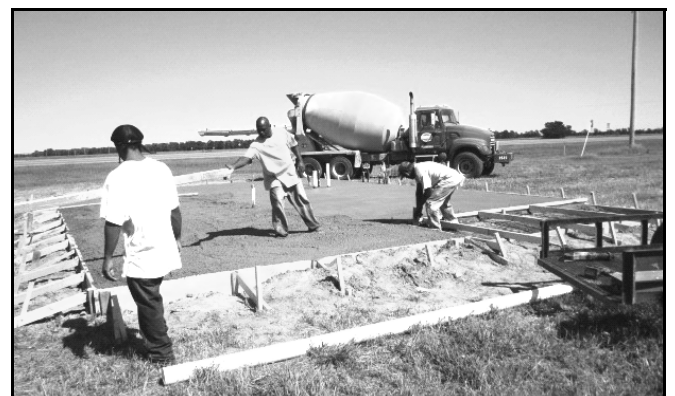
J.D. Smith (center) and friends pour slab for West Tallahatchie Habitat House #40!
